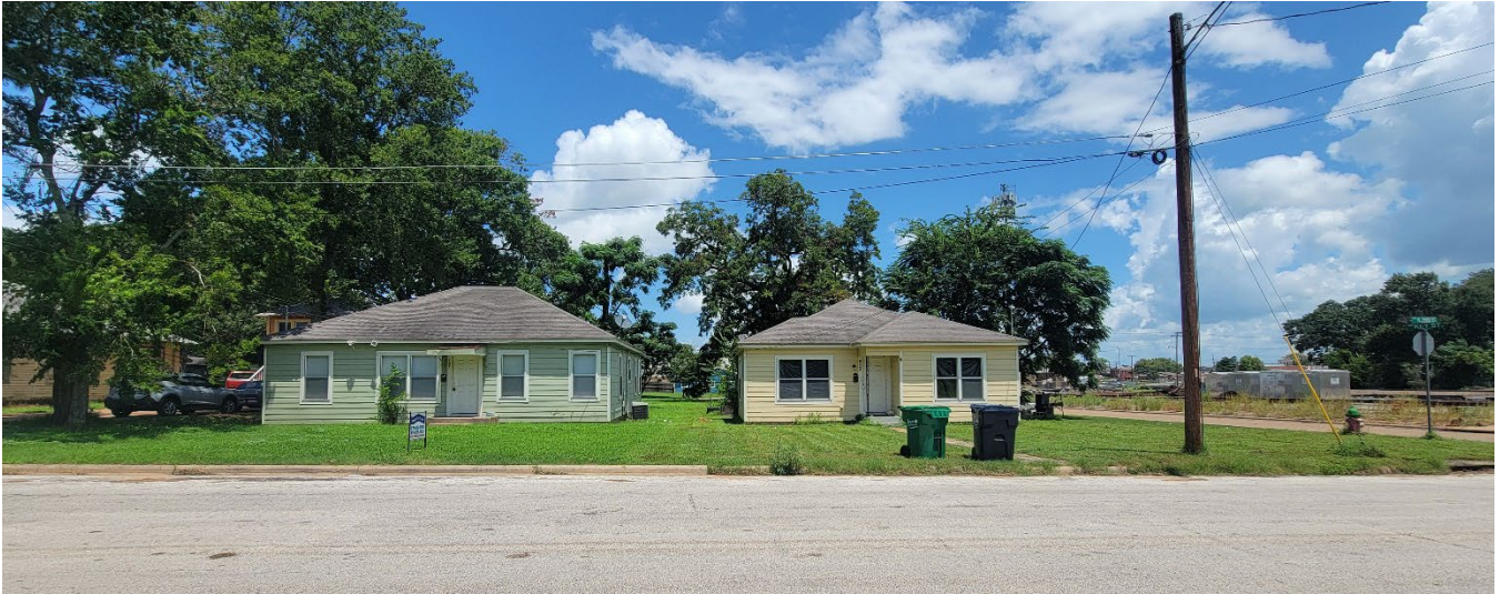
502 W. Third Street (Left) & 500 W. Third Street (Right)
