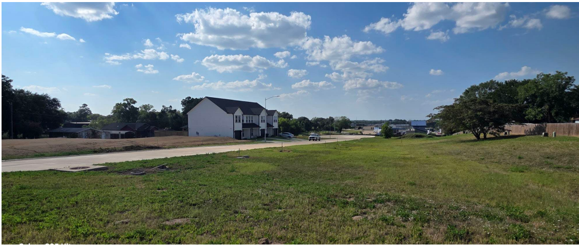
Ebenezer Lane to the northwest, across Clay Street. 30-unit townhome development. 3 units currently complete. Dirt work started on second building.
