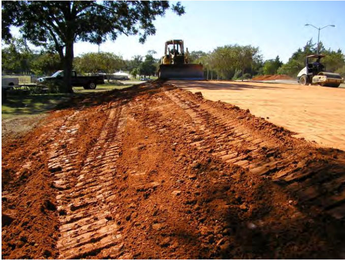
Pad work for the All Sports Building
