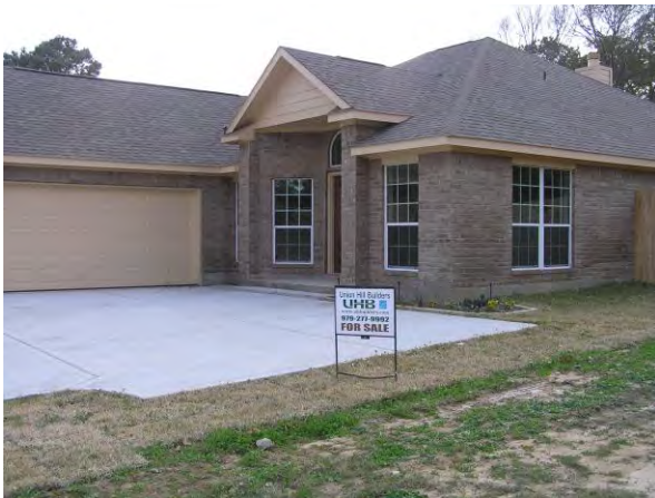
New residential construction on Ruth Circle
