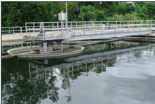
New Aeration Basin
