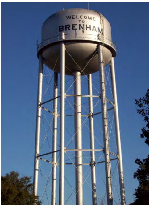
Church Street Tower
