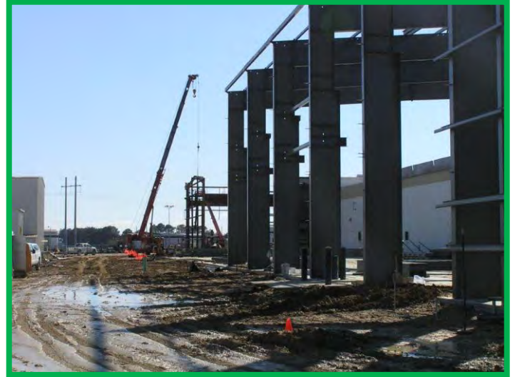
Valmont Light Pole Plant Expansion
