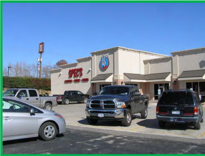
Completion of New Retail
