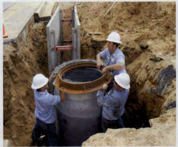
Manhole Installation
