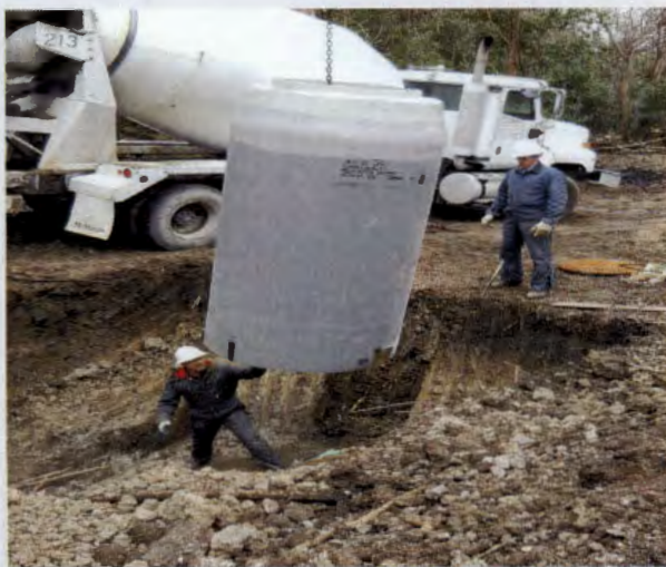
Manhole Installation
