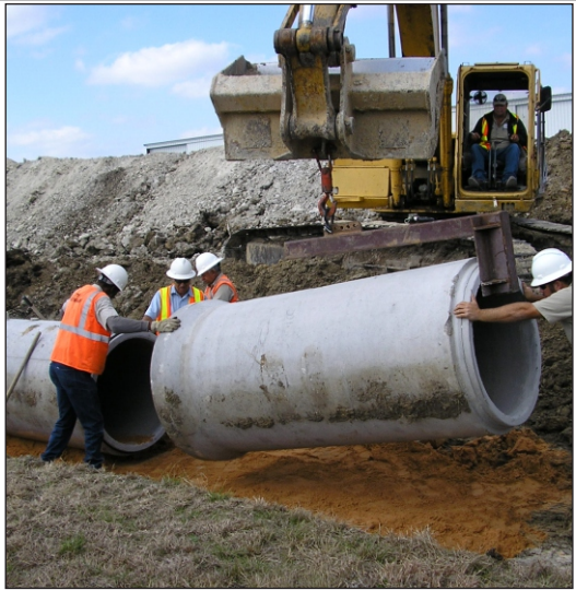
Installation of RCP culvert for erosion control.
