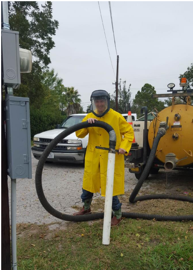
Sean Church Utilizing the Vac-Unit to Excavate Utility Line Locations
