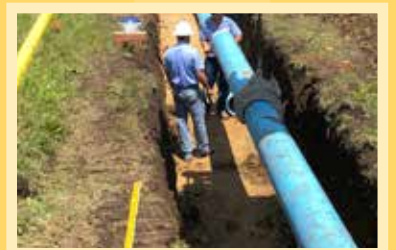
Water Install Baker Katz
