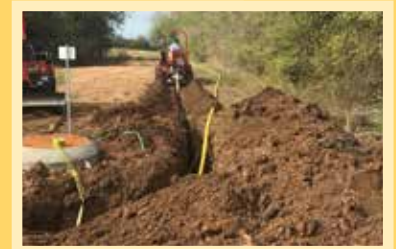
Gas Line Install Baker Katz
