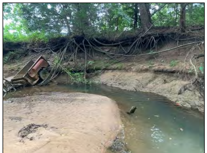
Photo 24: Upstream-facing view of truck and surrounding conditions.
