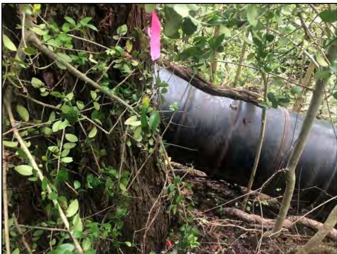
Photo 5: Upstream-facing view of the tank in creek near Transect 10.
