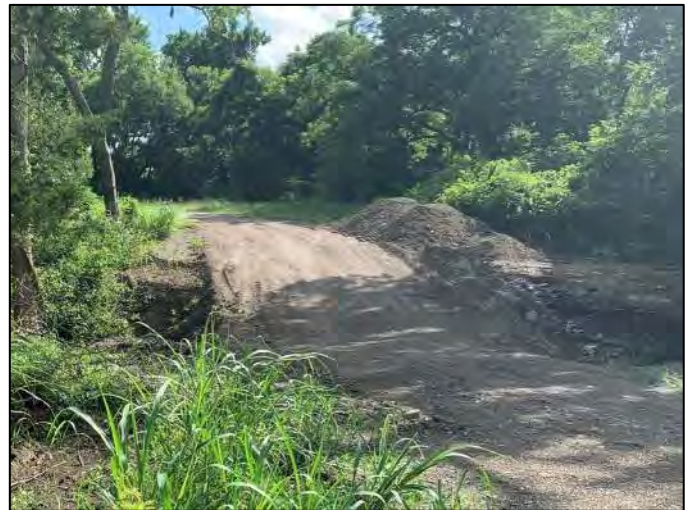
Photo 42: North-facing view of the dirt road crossing the culvert at the southern terminus of the Site.
