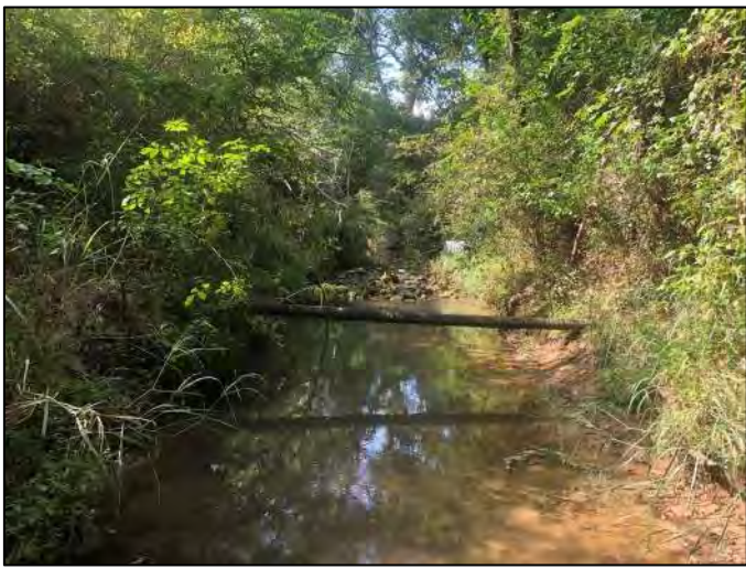
Photo 13: Upstream-facing of gas pipeline.
