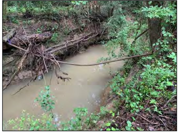
Photo 16: Upstream-facing view of remnants of a metal gate crossing the creek.
