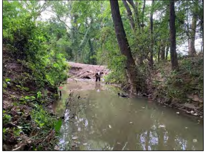
Photo 40: Downstream-facing view of southern dirt road and culvert.
