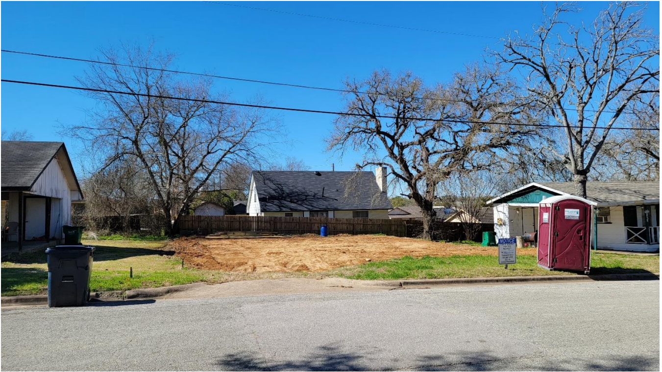
Subject Property – Being graded for foundation
