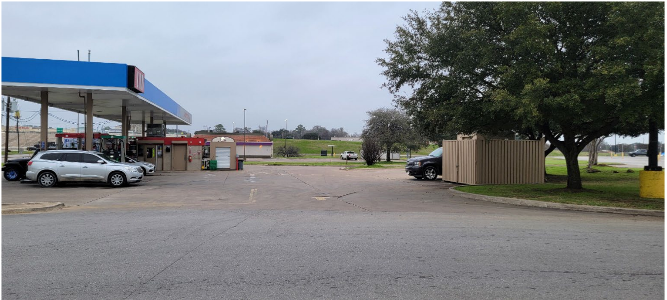
Convenience Store will be constructed in the southeast corner where the existing dumpster is located.
