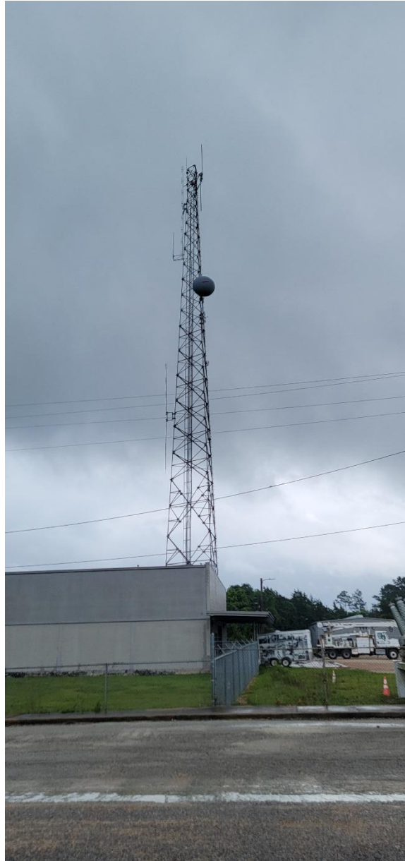
Existing 190-foot Communications Tower
