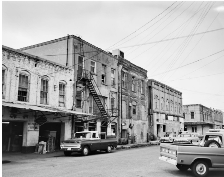
Figure 1 Fire Escape Stair – Commerce Street
