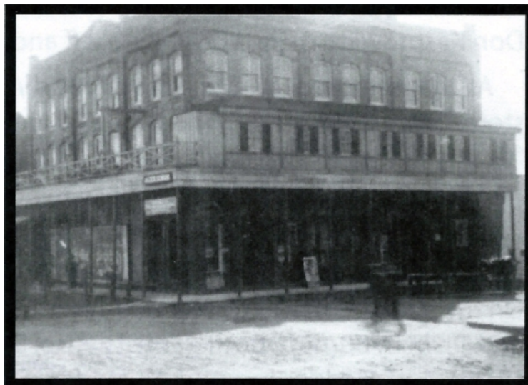
Figure 2 Brenham Opera House w/ Exposed Steel Columns, Balcony, and Canopy
