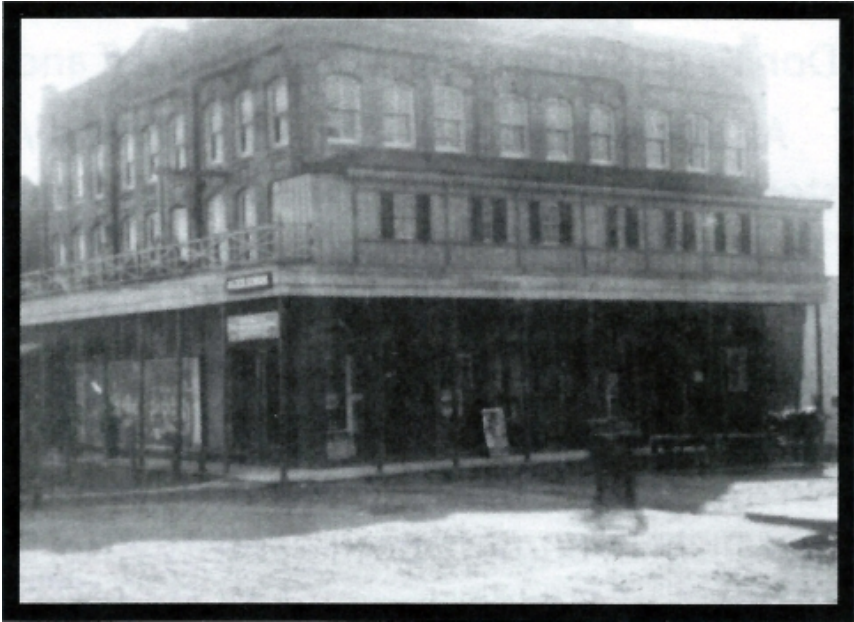
Figure 3 Historic Brenham Opera House with exposed steel column construction
