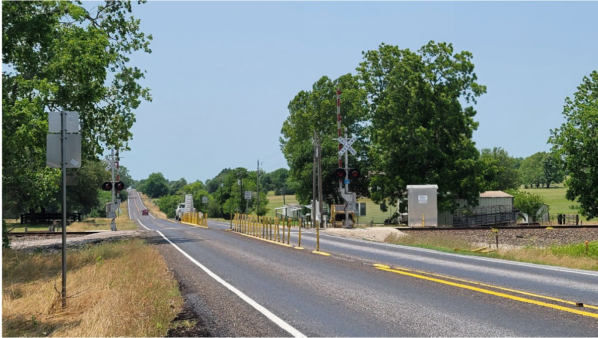
Looking west- City limits at railroad crossing
