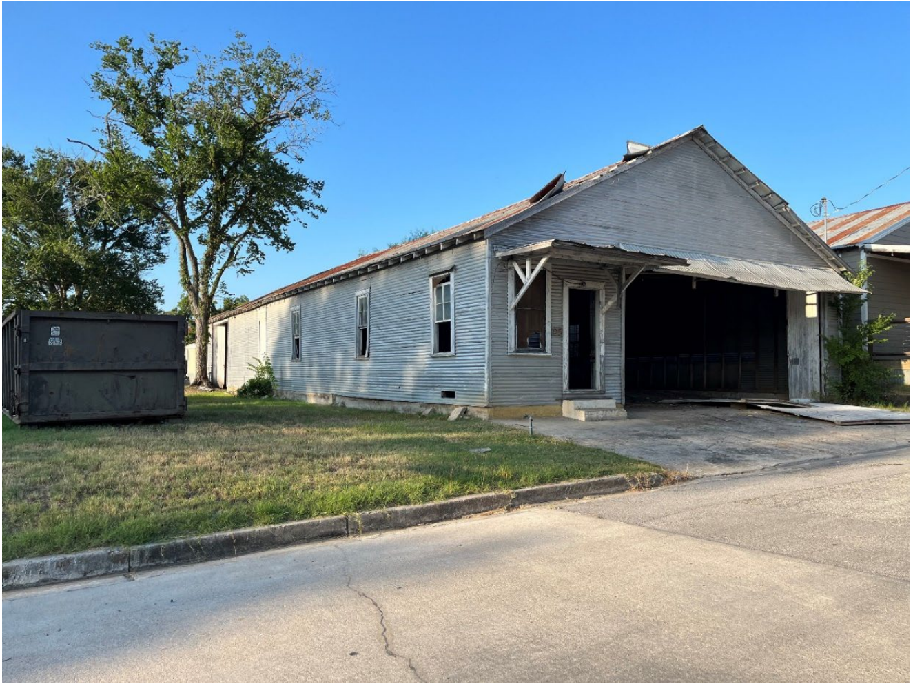
View of warehouse structure from corner of First Street at Park Street
