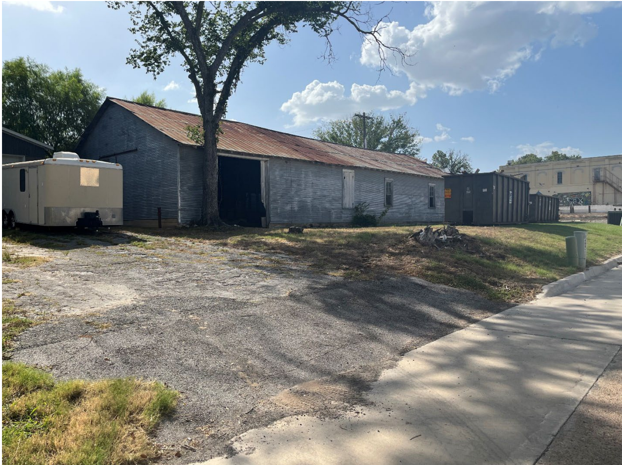
View of the back and side of warehouse from Park Street
