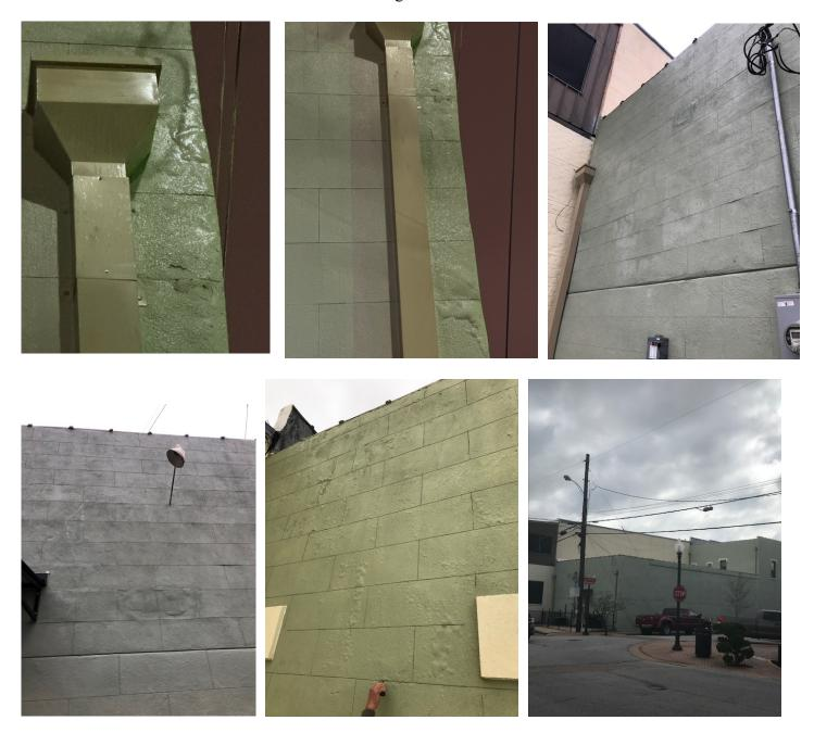
This second story wall causes the most damage inside the building when it rains. The water runs down this wall and enters the building at the first story roof/attic space where the first and second stories meet. The water collects in the attic space and comes into the offices below.
