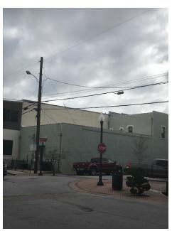
This second story wall causes the most damage inside the building when it rains. The water runs down this wall and enters the building at the first story roof/attic space where the first and second stories meet. The water collects in the attic space and comes into the offices below.
