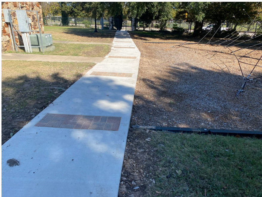
Sidewalk Repairs – Fireman's Park
