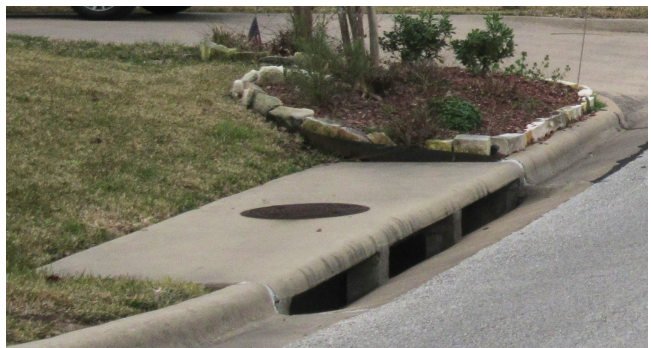
Stormwater runoff collection
