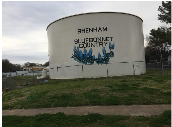
City of Brenham utility infrastructure.
