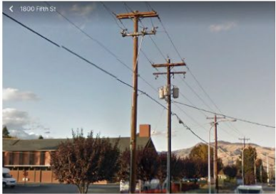
Upgrading existing neighborhood Distribution lines
