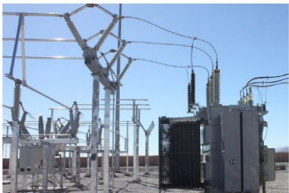
Adding neighborhood Substations
