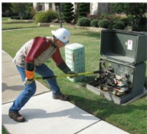
Upgrading existing transformers
