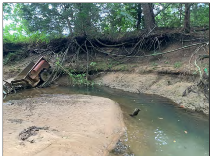
Photo 24: Upstream-facing view of truck and surrounding conditions.
