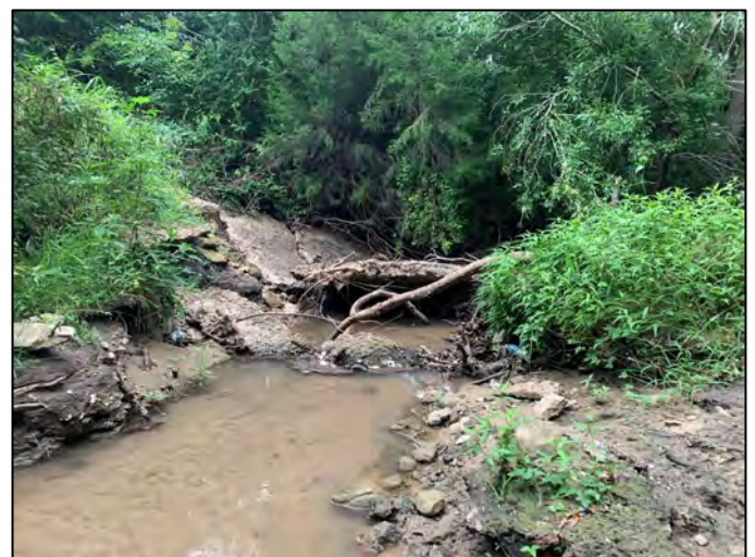
Photo 30: Downstream-facing view of creek and collapsed road.
