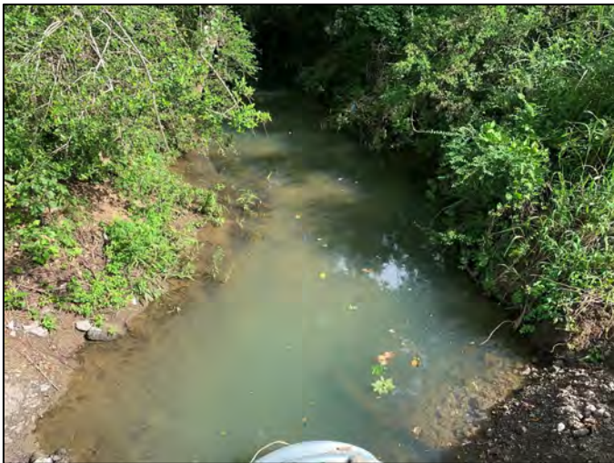
Photo 41: Upstream-facing view from dirt road crossing culvert.
