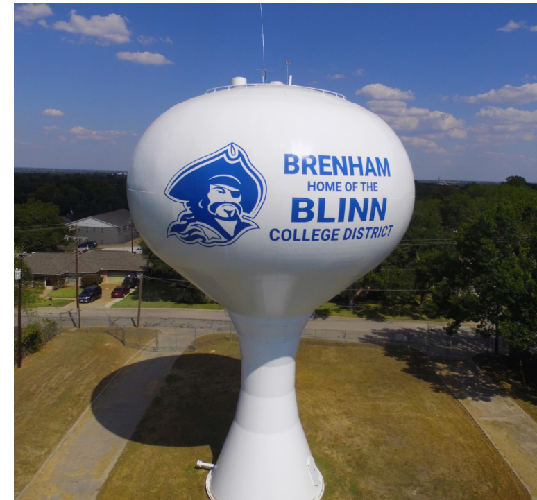
Atlow Elevated Storage Tank
