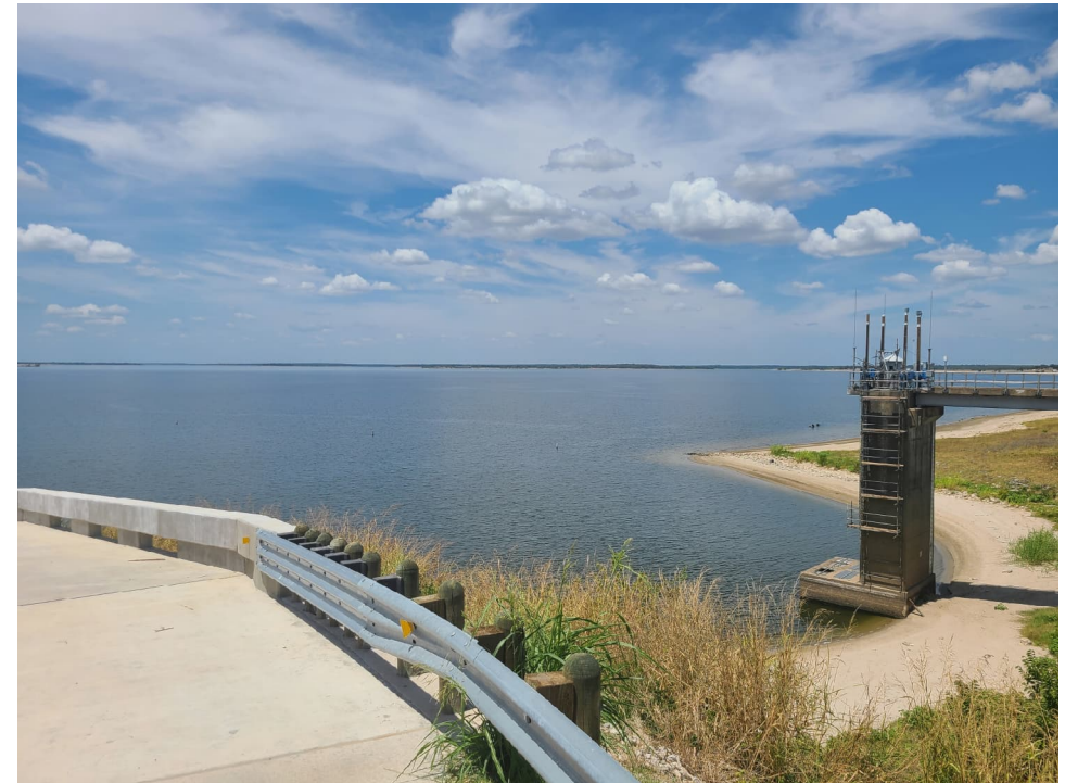
Lake Somerville Intake Facility
