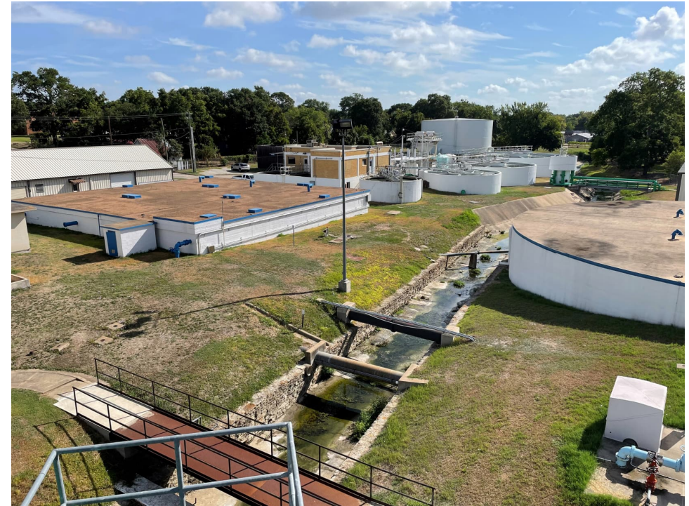
Surface Water Treatment Plant
