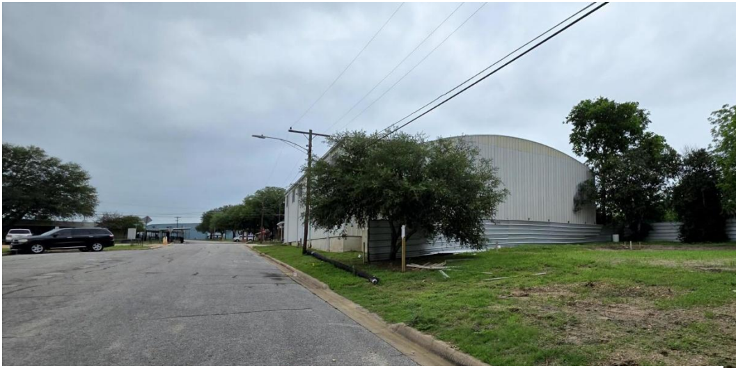
West Mangrum Street- Early Childhood Center on the corner of Mangrum and Kerr Street, with StanPac in the distance.
